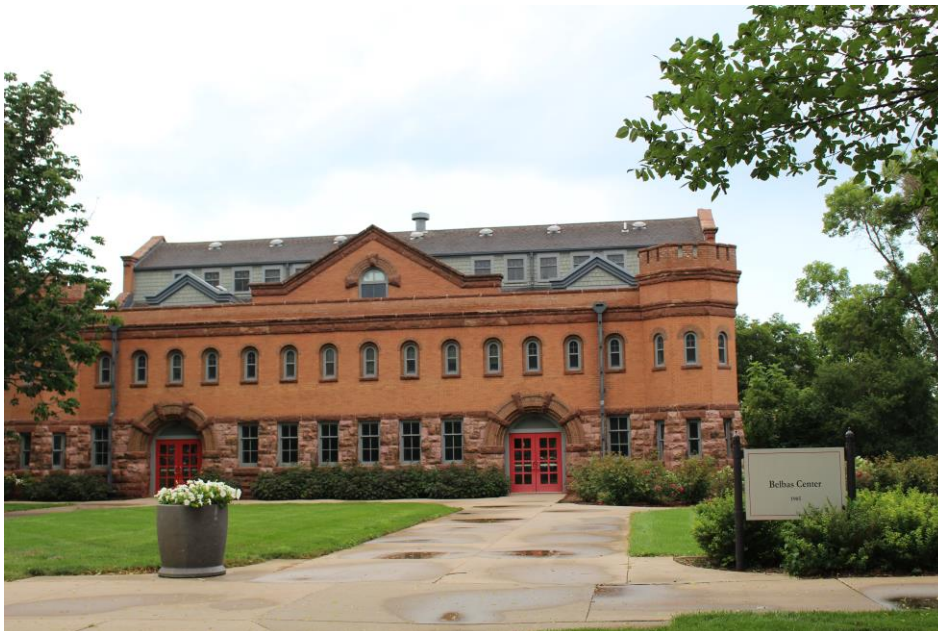
3. Armory/Gymnasium (Old), south elevation (camera looking north)
