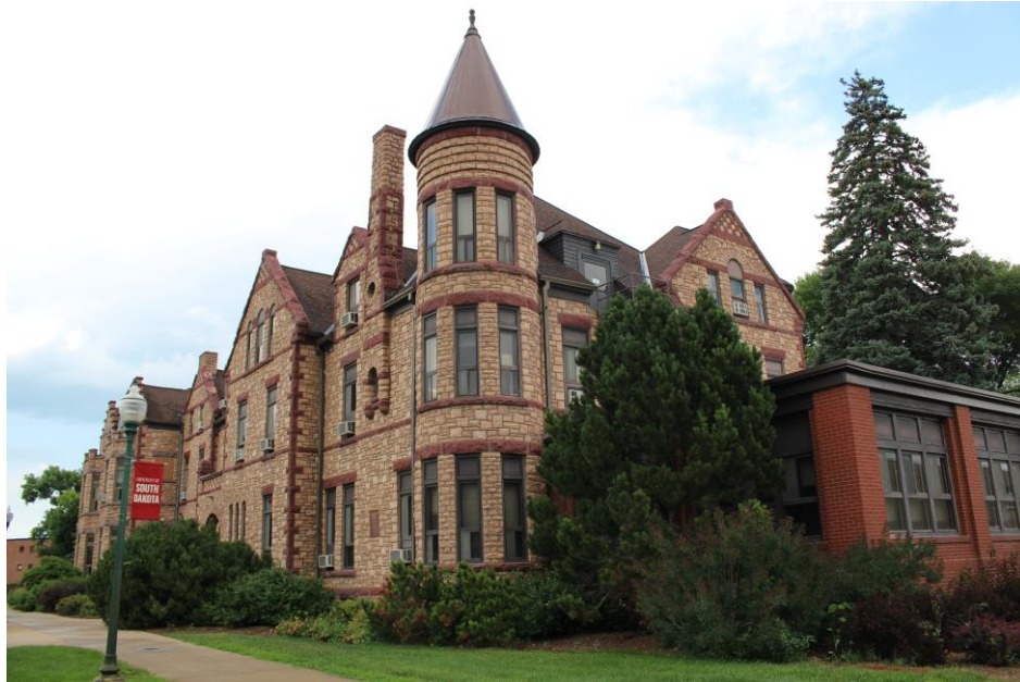
2. East Hall, south west corner (camera looking northeast)
