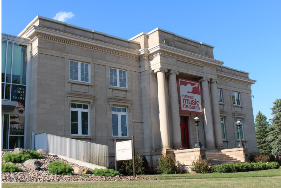
6. University Library, front (south) elevation (camera facing northeast)
