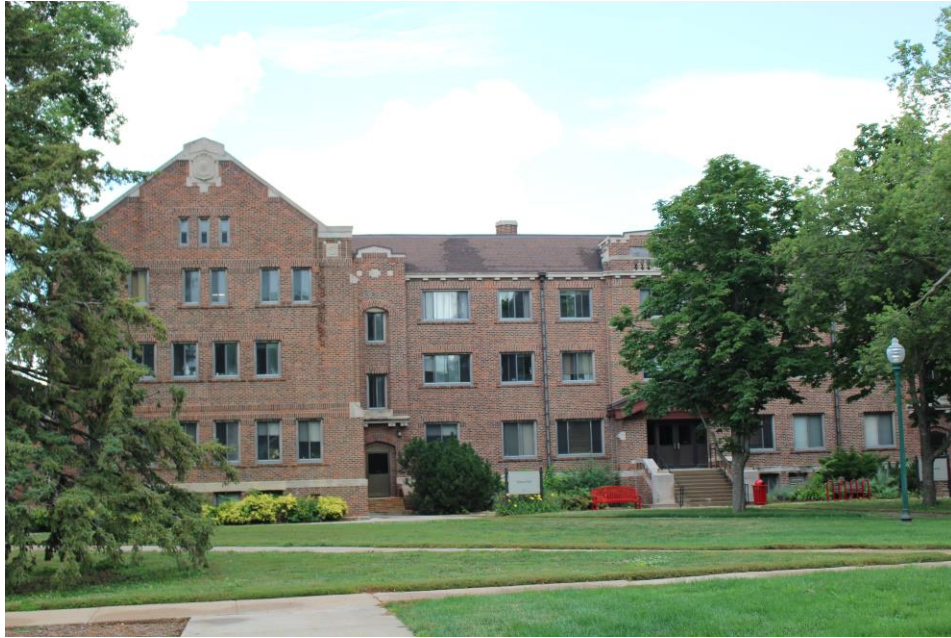
8. Dakota Hall, front (west) elevation (camera facing east)
