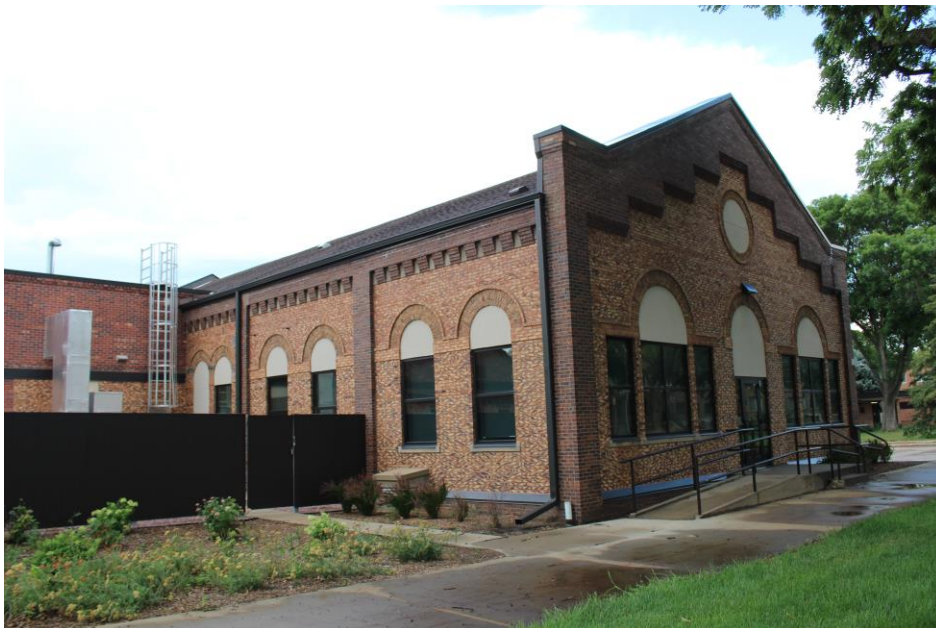
5. Old Power Plant, south and west wings, southwest corner (camera facing northeast)
